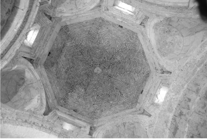
Fig. 3.3.23 Cloister vault of the Church of Yoldath Aloho at Ḥāḥ
